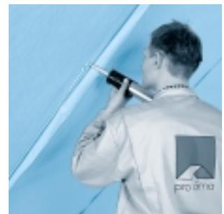
Turn the overlapping or connecting piece back again and press it to the piece below.
