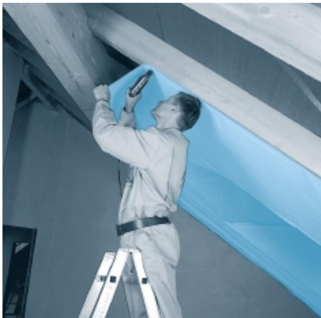
Attach the remaining piece of the strip after the paper has been installed: Lift up the piece, apply a line of adhesive, press down the strip and (in the case of wood or plaster) if necessary staple it to the surface underneath.
