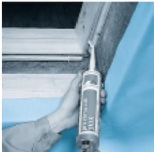
Attaching to rooflights
