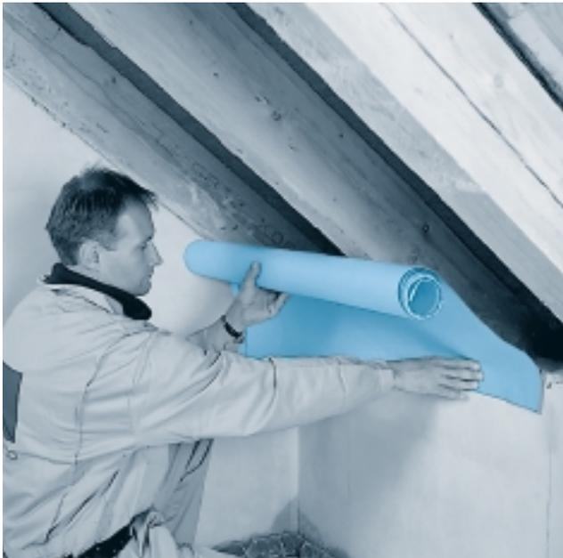
Roll up the pro clima paper tightly that it can be grasped in one hand. Start at the bottom rafter. Staple the free end to the bottom rafter or the rafter closest to the bottom rafter in one place. Then unroll the paper upwards along the structure until about 1m below the end of the rafter, straighten it out and attach it to the rafter.
