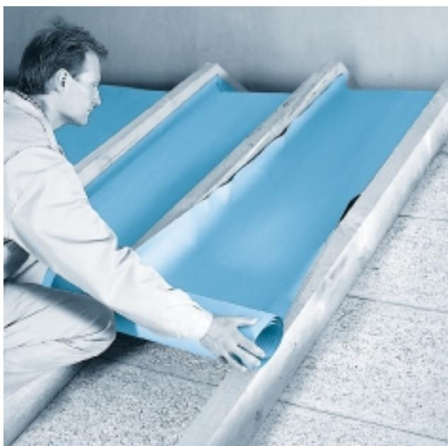
After the roof lathing and if necessary the old insulation have been removed, lay the appropriate pro clima paper parallel to the edge of the gable wall, i.e. from the top to the bottom, on the inside sheathing.
