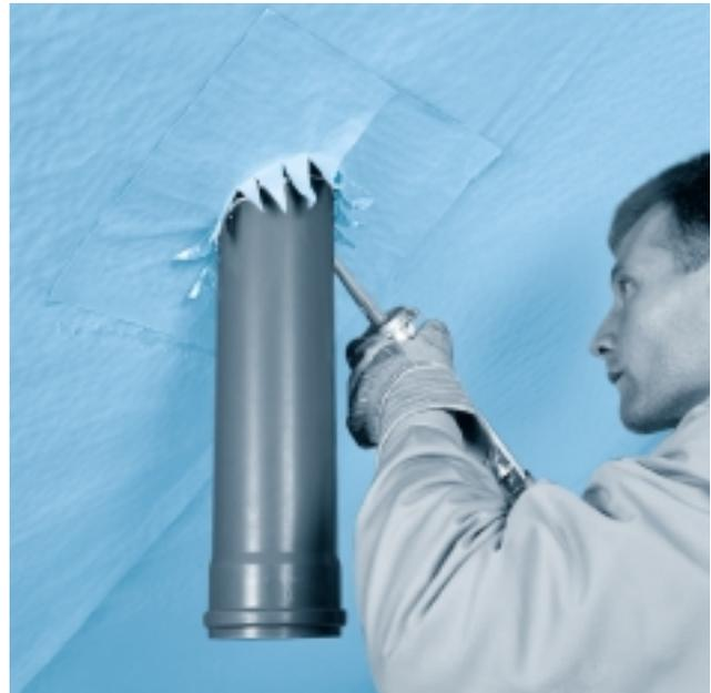
Then install the counter-sleeve also using pro clima COLL. Counter-sleeves are available for roof pitches of 15–25°, 25–35° and 35–45°
