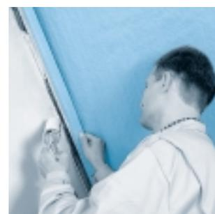
If the sub-surface is wood or plaster: staple the paper if necessary over the bonded join.
