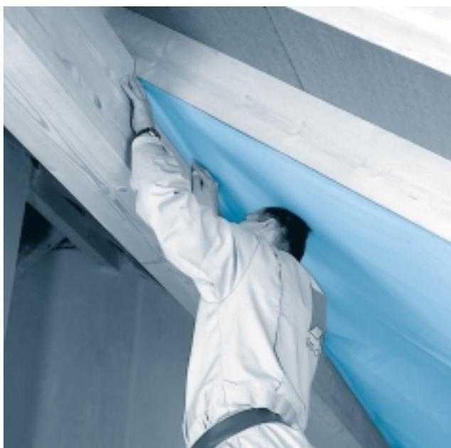
After the adhesive has dried any extra pieces of the paper can be cut away with a sharp carpet knife.
