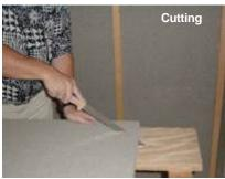
The cutting takes place with one cutting motion using the entire length of the blade.
