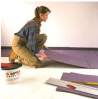
Leave a movement gap of 8mm from the wall. If the carpet is to be adhered to the HAPPY-STEP, the boards should also be glued to the substrate. To do so, apply a natural latex adhesive or double side tape to at least the four corners and middle of each board.
