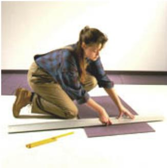
Always lay the HAPPY-STEP in a 'brick-like' formation re-using the off-cut from each run to begin the next (see diagram in pack). For best results install the HAPPY-STEP boards perpendicular (or at 45°) to the principal direction of the joints or pattern of the intended floor covering (it is preferable for the direction of the principal joints or pattern of the floor covering to be parallel to the wall containing the primary light source).
