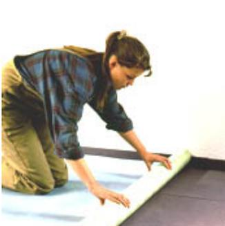
Adhere the carpet / cork tiles to the HAPPY-STEP boards using a suitable adhesive (e.g. *Holzweg natural latex flooring adhesive* by Construction Resources).
