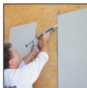
Application of joint adhesive
