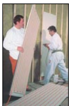
Assembly of Modular Panels
