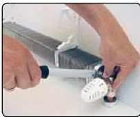
Connecting supply pipe
