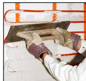
Application of Eco-Heating Plaster
