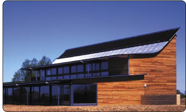
The ES Solar Roof is ideal in public, commercial and industrial building applications. Here showing its use in the sports facilities of Great Notley Discovery Centre, Essex (photo © Sue Barr)
