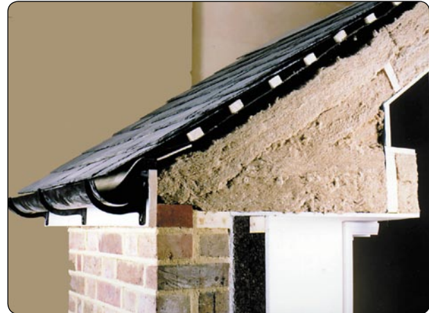
This cross-section demonstrates the use of flax insulation batts to insulate the roof of a solid brick construction. 200mm of flax has been used between ceiling joists and between the rafters.
